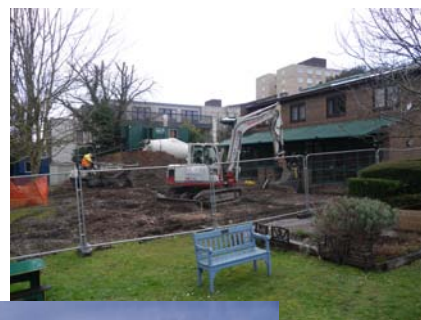
Feb 2014: digging the foundations
