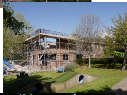
May 2014: roof joists fitted
